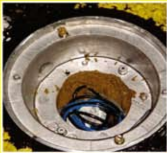
Installation of landing lights
