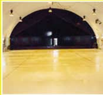
Aircraft hangar floorings
