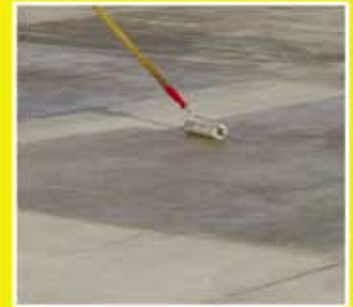
Protection with in surface sealers
