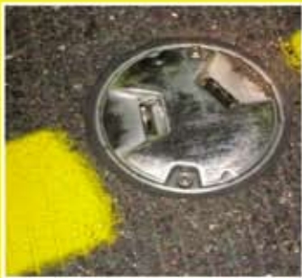
Installation of landing lights
