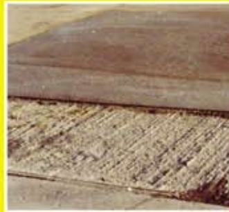
Patch repairs to pavements
