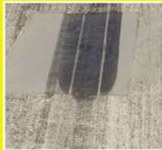
Patch repairs to pavements
