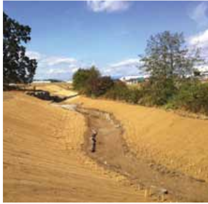
The Reay Creek Remediation Project as of October 2, 2012.
