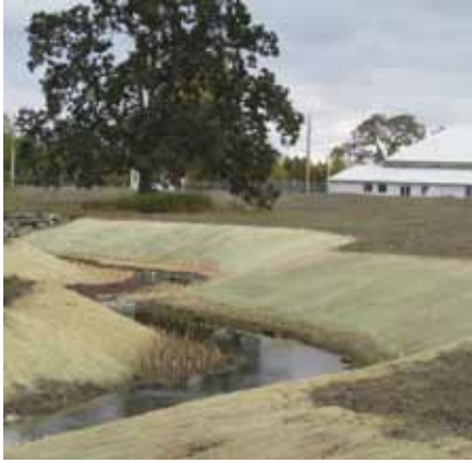
The Reay Creek Remediation Project as of September 2, 2012.
