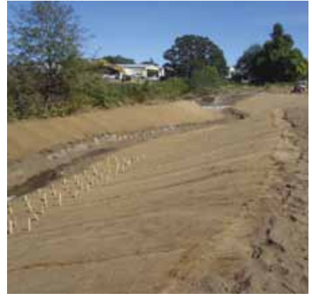
The Reay Creek Remediation Project as of October 3, 2012.
