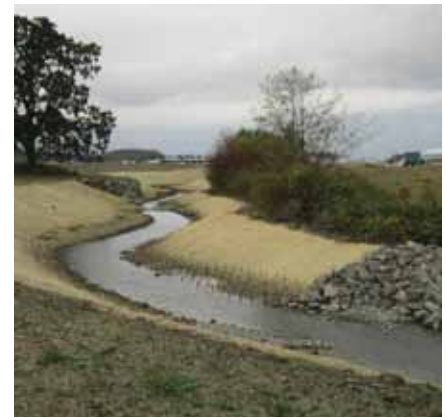
The Reay Creek Remediation Project as of September 1, 2012.
