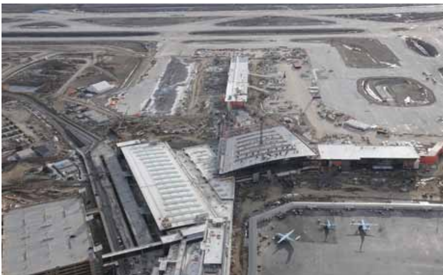
About 183,000 square metres will be added to the Calgary International Airport.
