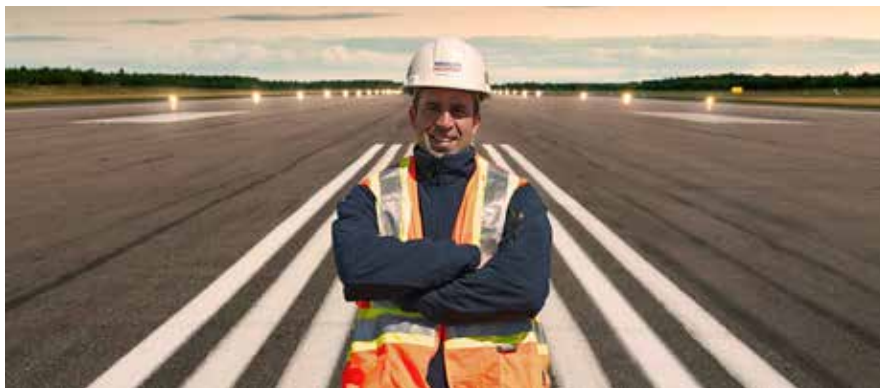
Crews need to be ready for the unexpected and able to troubleshoot problems quickly, because when you're working on a live runway, there is no margin for error.
