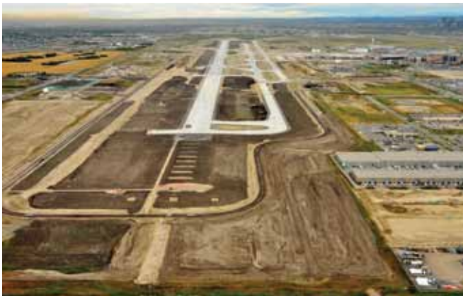
The YYC's $620-million runway project will double the airport's airfield capacity.
