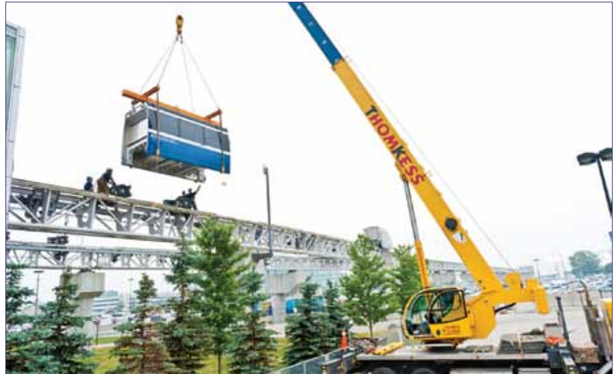
Installation of the platform door for Automated People Movers LINK 7th cabin project.
