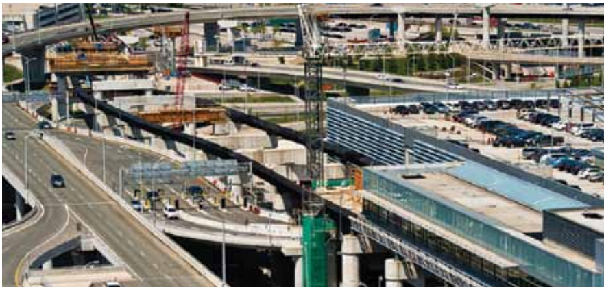
Air Rail Link construction, as seen from the Terminal 1 Apron Tower.
