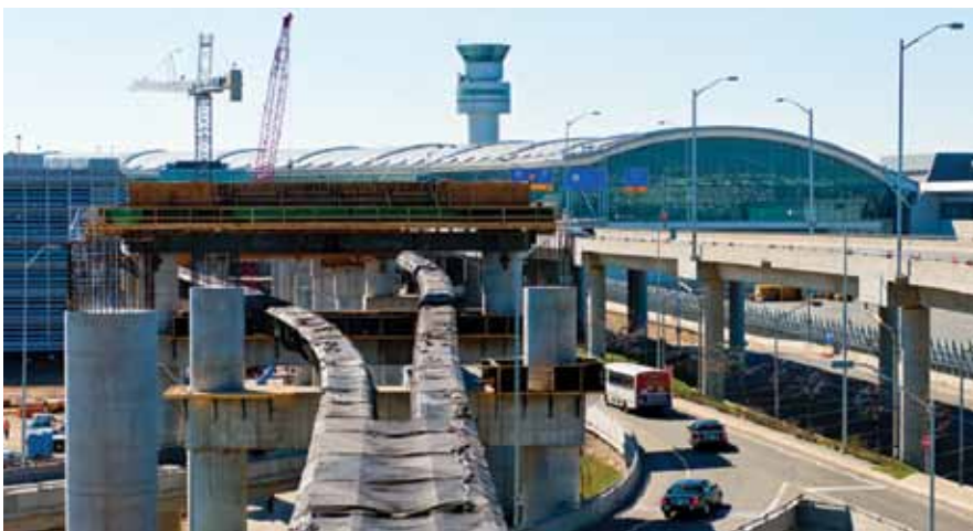
Construction of Air Rail Link pier bents.
