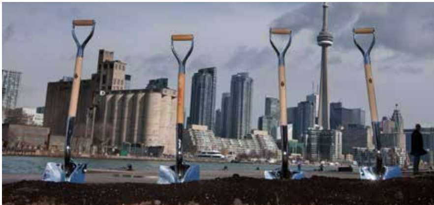
Preparing to break ground on the new pedestrian tunnel to Billy Bishop Toronto City Airport in 2012.
